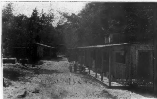
Some of the Employees Quarters
